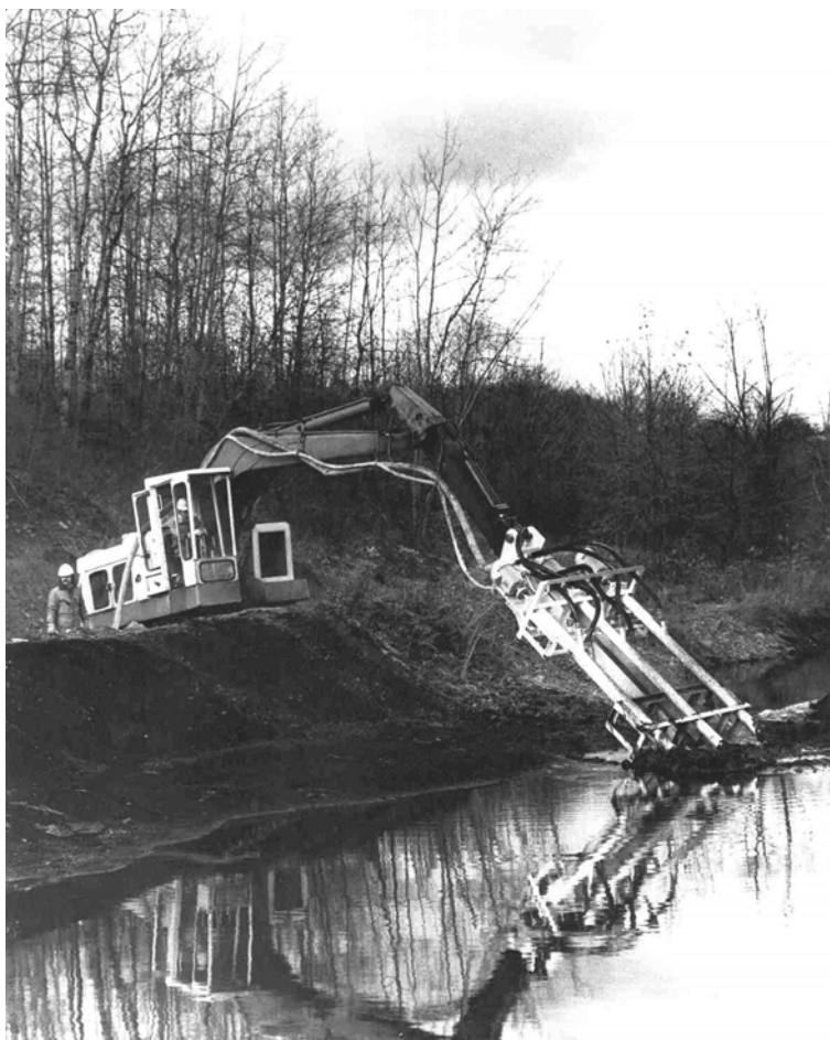
FIGURE 13.3 In situ mixing with backhoe-mounted rake injector.
