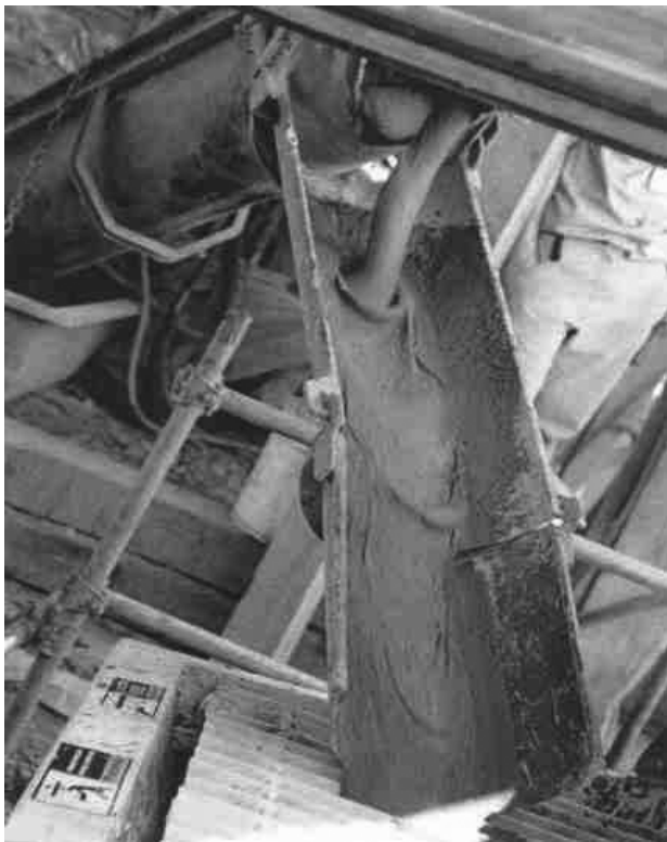
FIGURE 13.16 Tank 17 zero-bleed fill being discharged into the pump for Case Study #4
