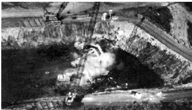
FIGURE 13.2 In situ mixing with backhoes.
