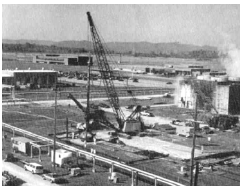
FIGURE 13.5 Photograph of actual in situ mixing with an auger system.
